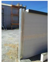
**Step 8 - post capping installation**Apply liquid nails underneath the post capping. Place the capping over the post and press down by hand then level the post top
